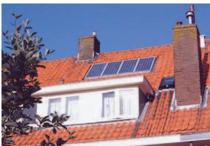
Example of a solar station with four 120Wp solar panels, suitable for Soladin peak capacity: 480Wp. Energy saving, depending on usage, up to 12%.
