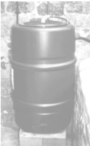
**1. The Rain Water Butt** - This collects rainwater from the roof via a *downpipe diverter* which fits onto our drain pipe. The butt houses a *submersible pump* on an extended leg attached to the lid. When the pump shuts off, all the water in the pipe back flushes cleaning the filter and ensuring that there is no water left in the supply pipe that could freeze. The butt also contains the *low level cut-off float switch* which activates to prevent the pump running dry.
